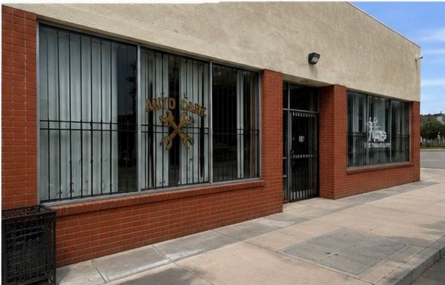
BEFORE – EXISTING CONDITIONS
