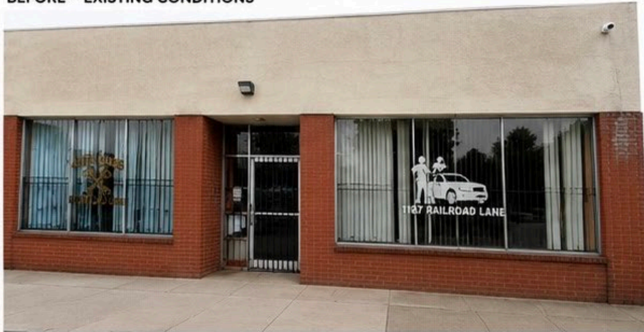
BEFORE – EXISTING CONDITIONS
