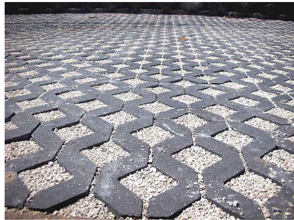
B EVA PAVING GRAVEL FILLED TURF BLOCK
