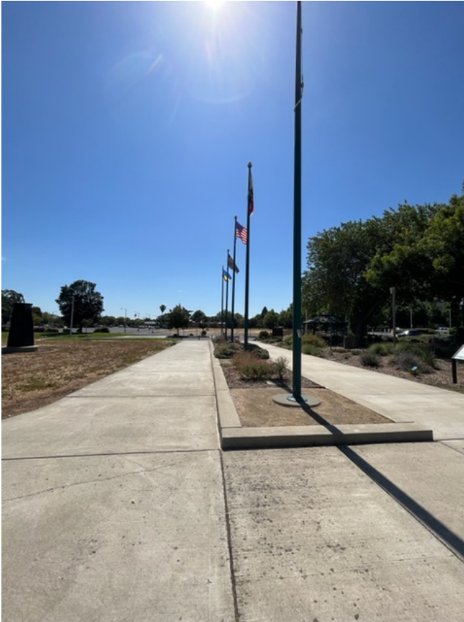
Existing flag poles along south side of project site boundary – to be removed and relocated to front of City Hall (location to be determined by City Manager).
