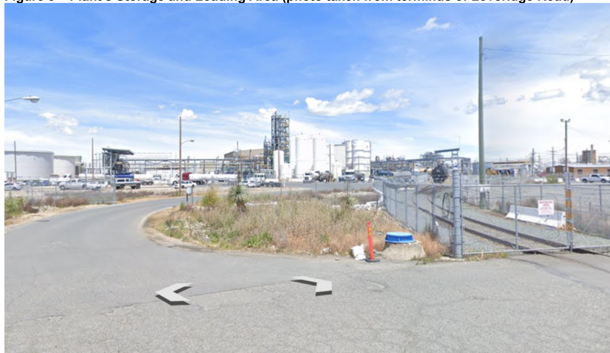
Figure 3 – Plant's Storage and Loading Area (photo taken from terminus of Loveridge Road)
