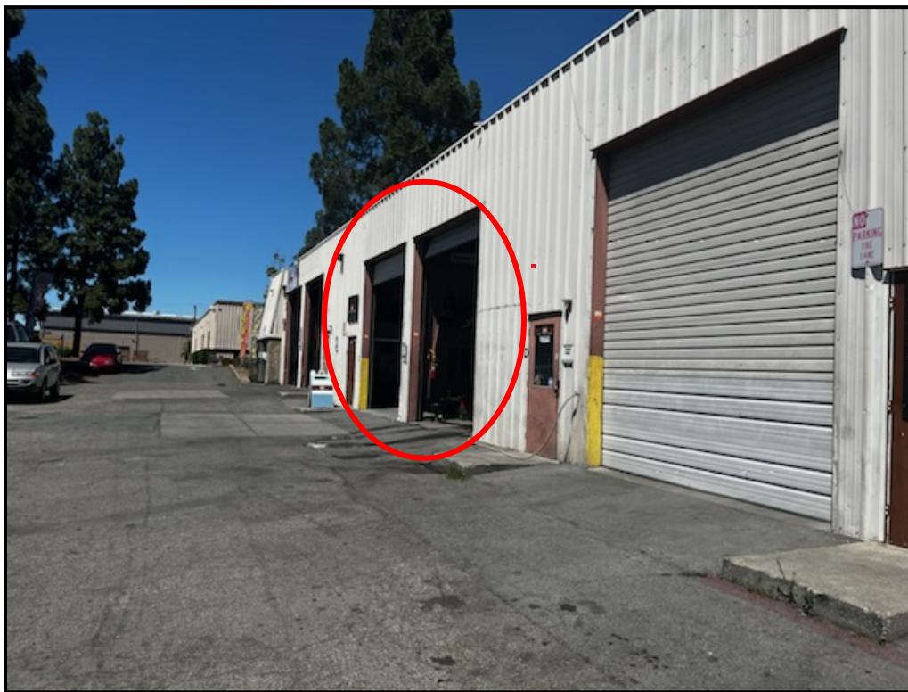
Fig. 1 Front of Warehouse Building Looking North from Project Site toward Garcia Ave
