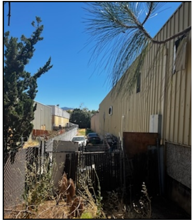
Fig. 5 – East Rear Yard of Warehouse
