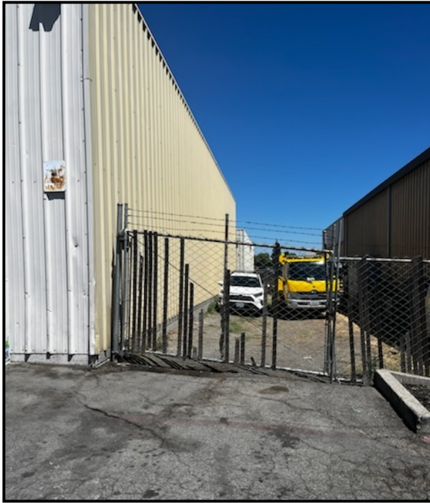
Fig. 4 – South Side Yard of Warehouse
