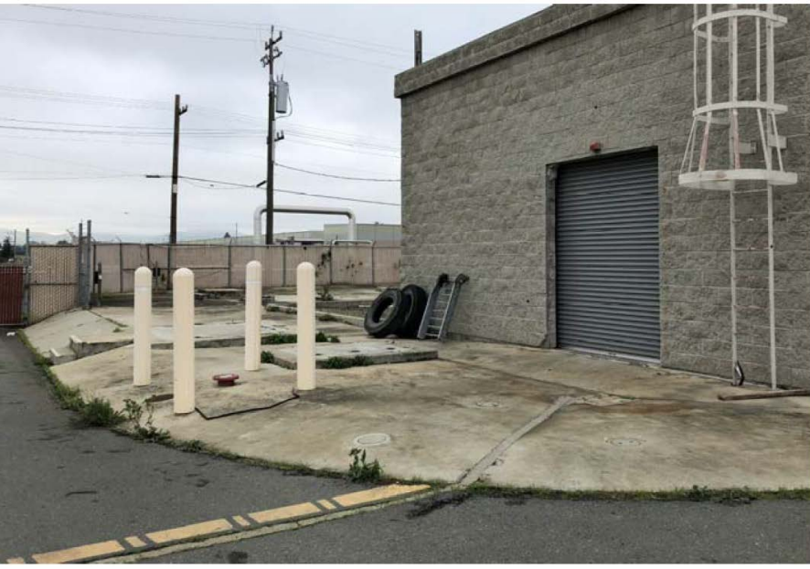
CORNER OF ROAD INSIDE 6
