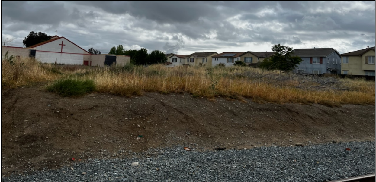
Above: View of Project Site from Union Pacific Railroad looking north toward Hamilton Memorial Church (to remain) and Central Ave
