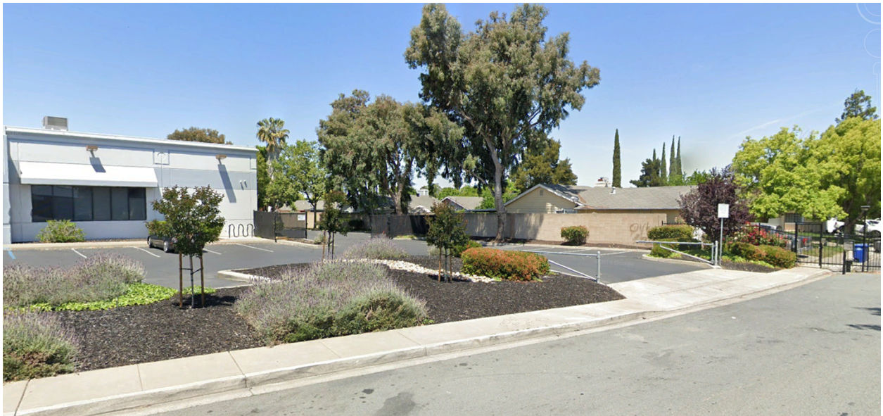
Photo 2: Looking north towards across Newport Drive at project entry and Stone Harbour Residential Subdivision
