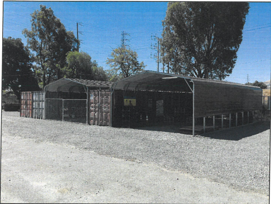
Carport & Storage Containers
