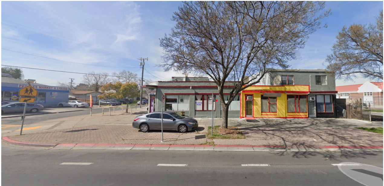
Harbor Street Frontage
