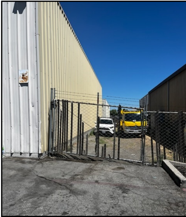
Fig. 4 – South Side Yard of Warehouse
