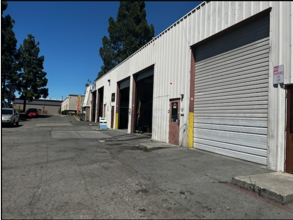
Fig. 1 Front of Warehouse Building Looking North from Project Site toward Garcia Ave
