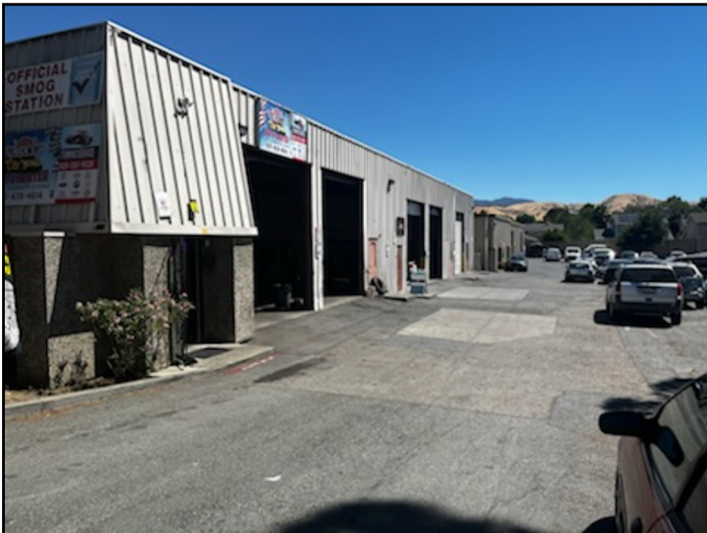
Fig. 2 – Front of Warehouse Building Looking South from Garcia Ave Driveway Entrance to Property
