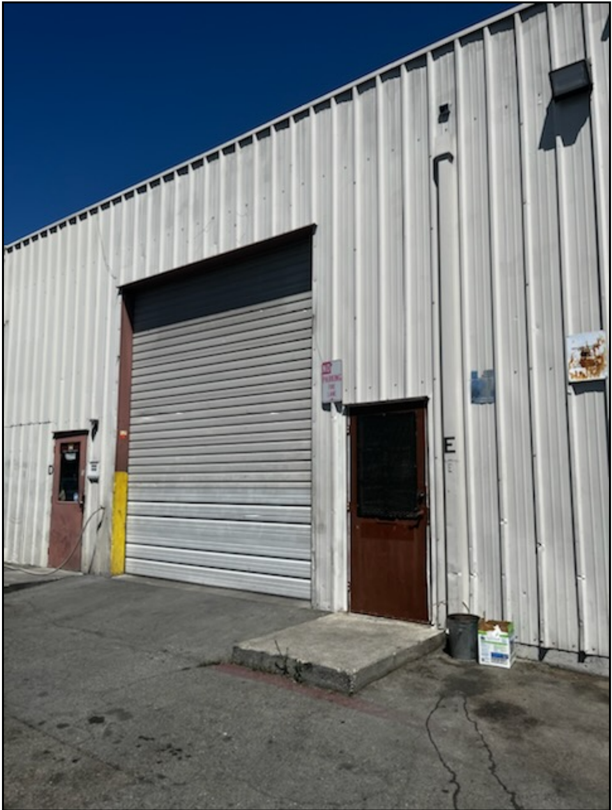
Fig. 3 – Suite E Vehicle and Pedestrian Entry Looking West from Parking Lot at Front of Warehouse Building
