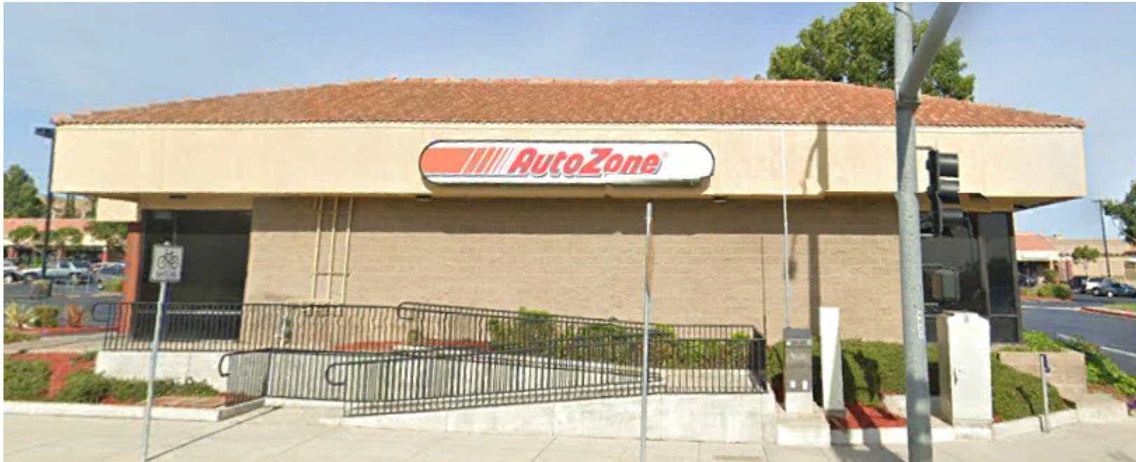
Auto Zone signage looking west.
