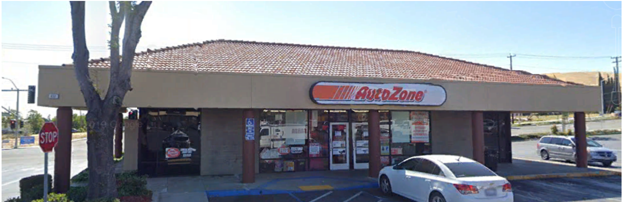
Auto Zone signage looking east.
