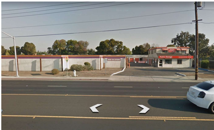
Figure 2: Existing storage and office/apartment building, facing north
