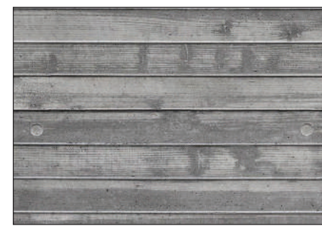
4 BOARD FORM CONCRETE
