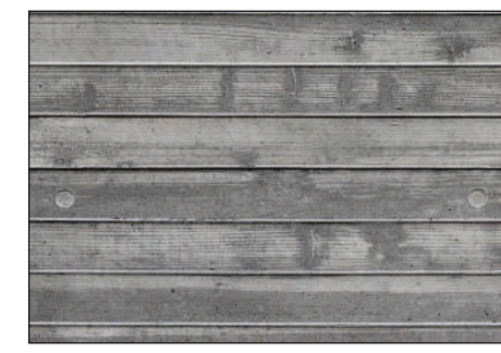
4 BOARD FORM CONCRETE
