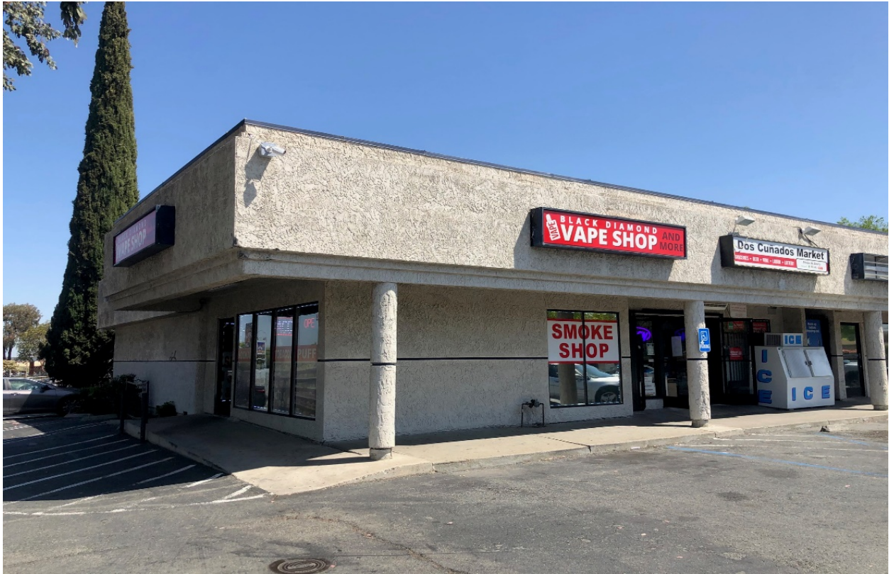
View of the southwest corner of the shopping center
