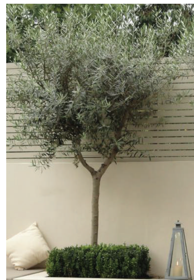
2 STUCCO WALL W/ PAINTED WOODEN SLAT PRIVACY SCREEN
