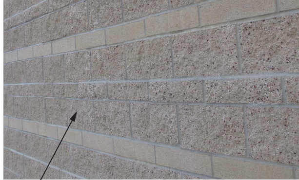
ANGELUS BLOCK - PLACER CREEK SPLIT FACE USE: EXTERIOR CMU BLOCK
