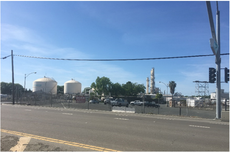
Figure 5: View west from Loveridge road
