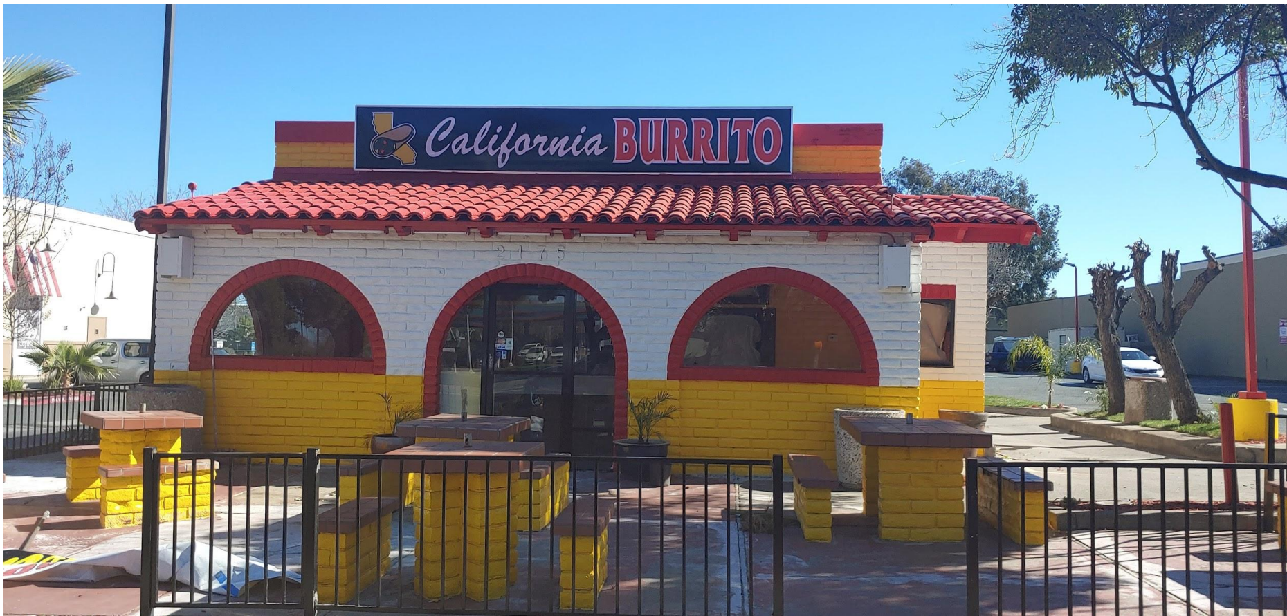
2175 Railroad Avenue Front Elevation
