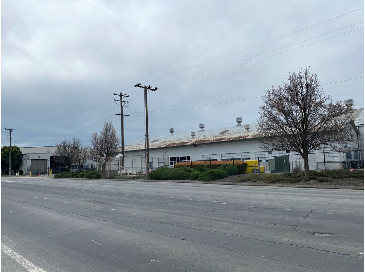
Above: Existing Transfer Station Building as viewed from Loveridge Road looking southwest
