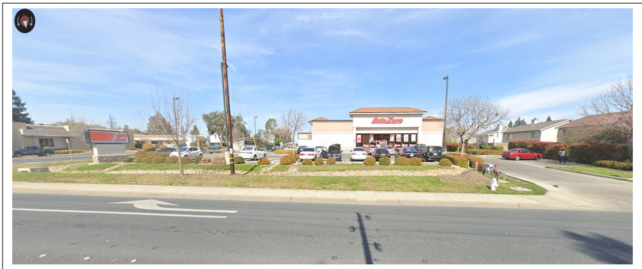
Fig. 3 (below) – Existing AutoZone Building, Frontage and Signage Looking North from East Leland Rd.
