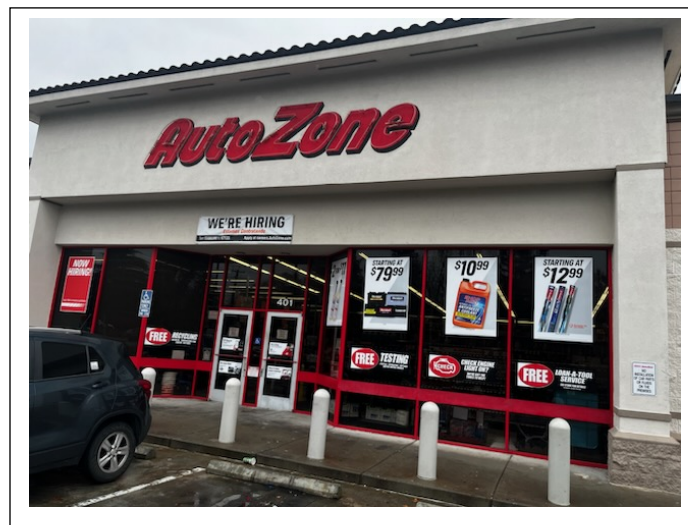
Fig. 6 (above) – Closeup of Existing Storefront/Main Entry Looking North from East Leland Rd.
