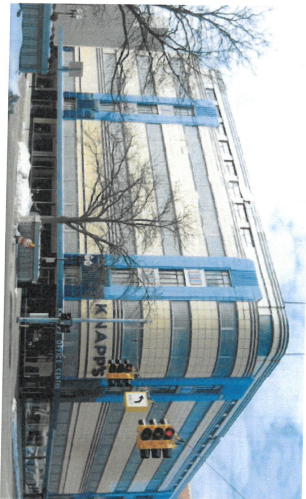
[7] (a) J.W. Knapp's Department Store, built 1937-38, in Lansing, MI, was constructed with a proprietary material named "Maul Macotta" made of enameled steel and cast-in-place concrete panels. Prior to its rehabilitation, a building inspection revealed that, due to a flaw in the original design and construction, the material was deteriorated beyond repair. The architects for the rehabilitation project devised a replacement system (b) consisting of enameled aluminum panels that matched the original colors (c). Photos and drawing (a-d): Quinn Evans Architects; Photo (c): James Haefer Photography.
