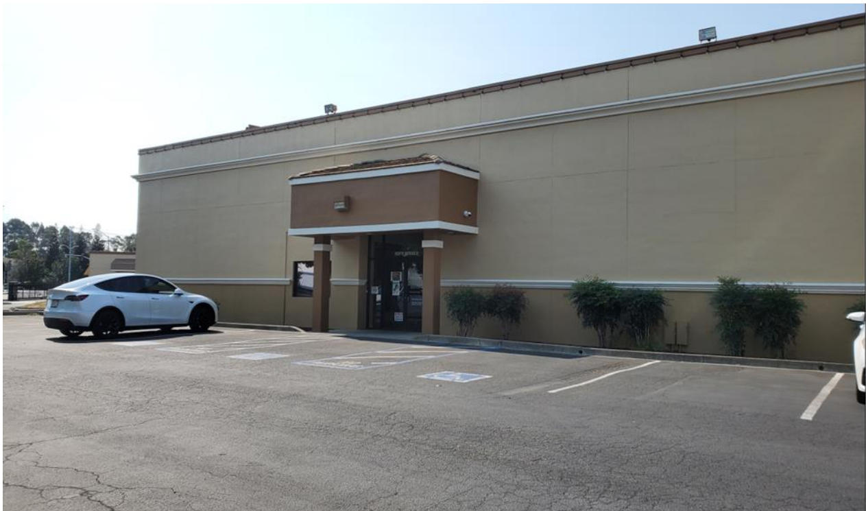
APN 088-570-014, facing south (closest building elevation adjacent to playground) Main Building: sanctuary, café, multi-purpose room and classrooms
