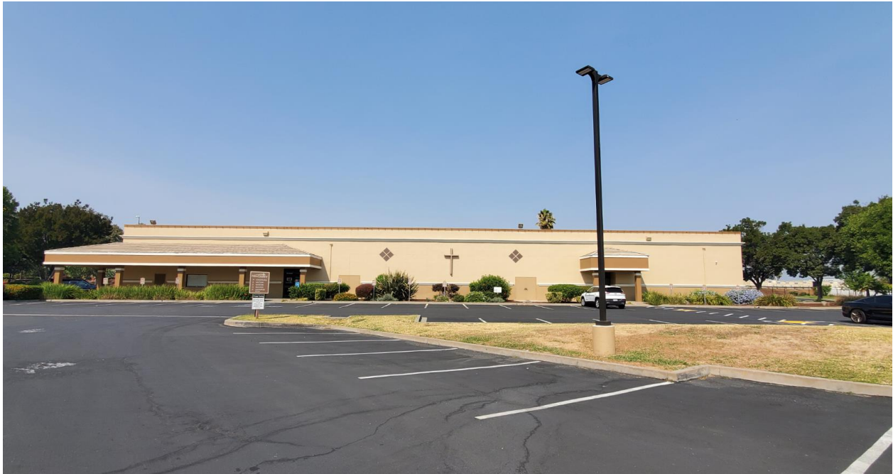
APN 088-570-014, facing west Main Building: sanctuary, café, multi-purpose room and classrooms
