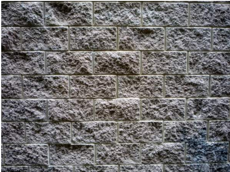
8" Split Face CMU Install Image
