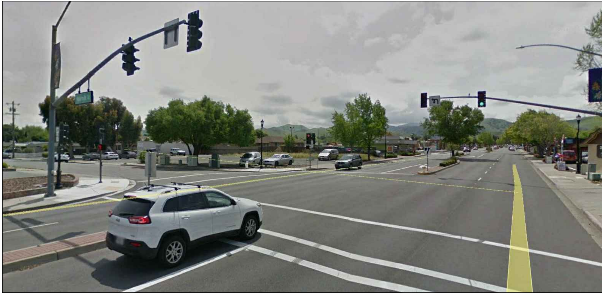
P002 LOOKING SOUTH
