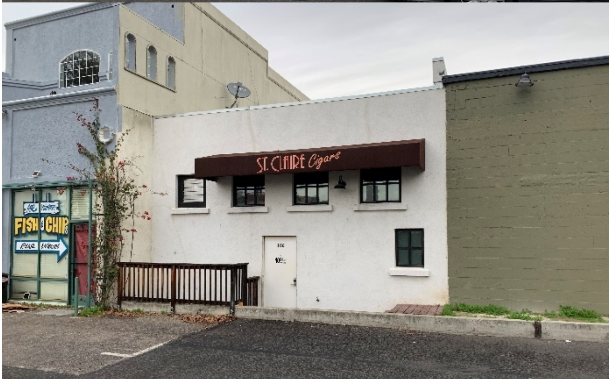
Fig. 1: Front façade along E. 4 th St.
