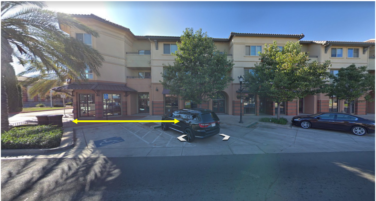
Figure 4: Eastern façade of tenant space, showing main entry point and adjacent commercial tenant spaces and residential units above. The yellow arrow identifies the general street frontage of the tenant space.
