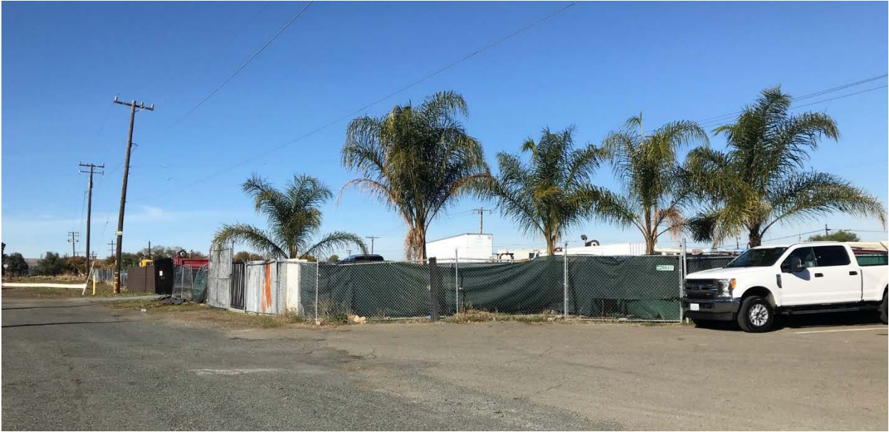
Above: View of Yard 2 looking west from N. Parkside Drive
