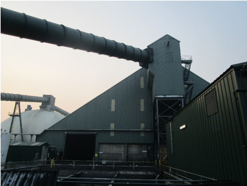
Photos of existing buildings on site:
