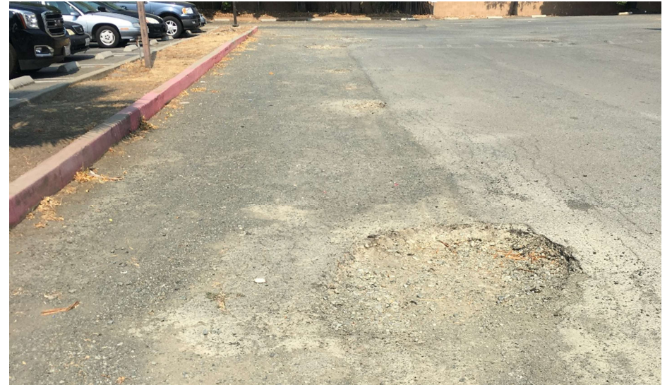
Figure 4: Existing drive aisle to be repaired.
