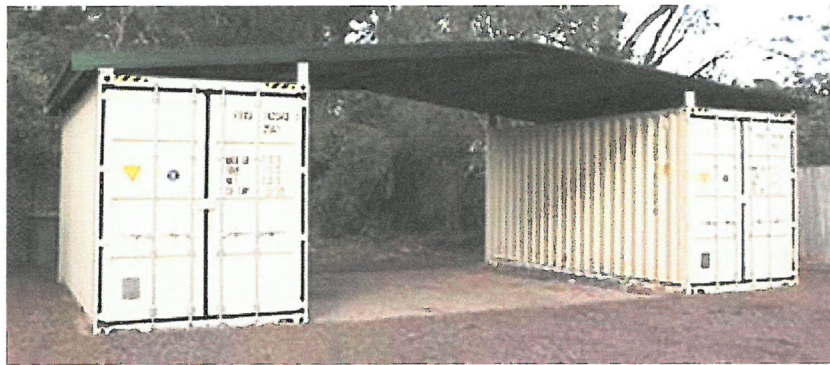
Family Room (temporary) roof between two storage containers (20'x20')
