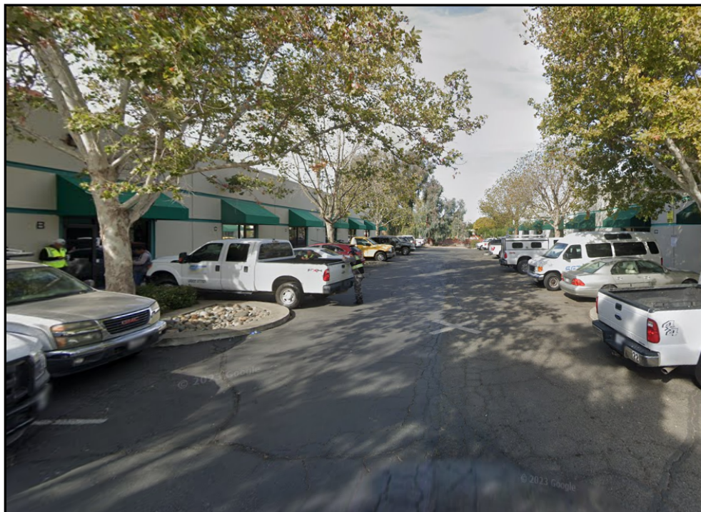
Fig. 2 (above) Front of Warehouse Building Looking West from Garcia Ave toward shared Parking Lot between 510 Garcia Building (on right) and 520 Garcia Building (on left)
