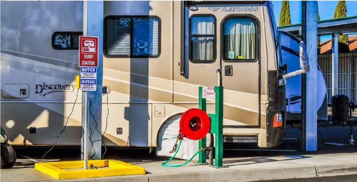
Typical Dump Station for customers
