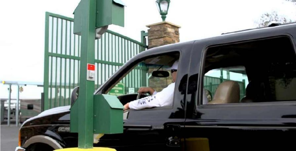
Typical Gate Entry and Keypad
