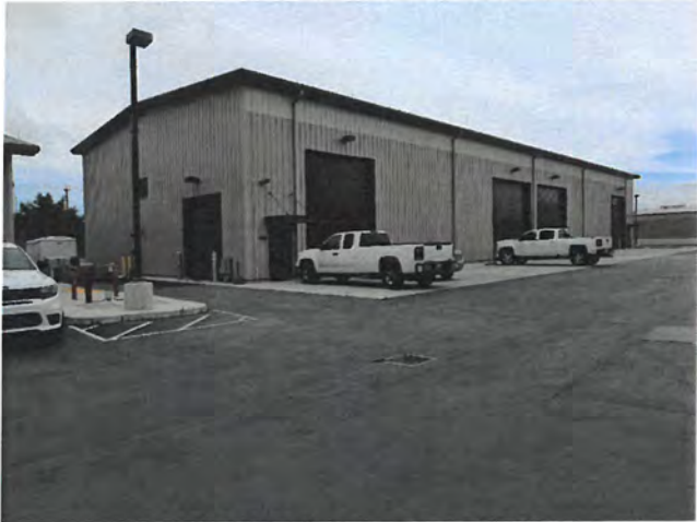
EXISTING NORTH ELEVATION- NO SCOPE OF WORK
