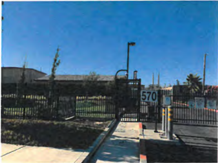
VIEW OF ENTRY FROM WEST 10TH STREET
