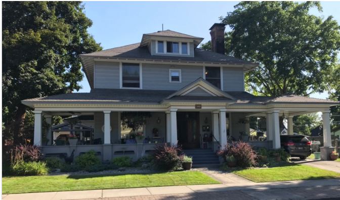
Example of Multiplex Small
