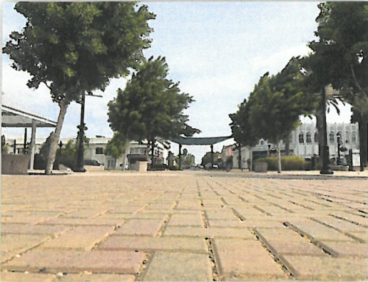
John Buckley Square permeable pavement
