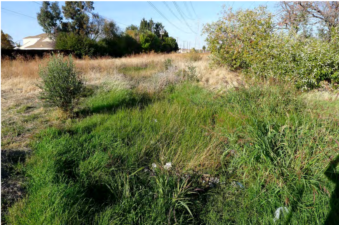
Surface drainage below culverts, looking N (11/17/14)
