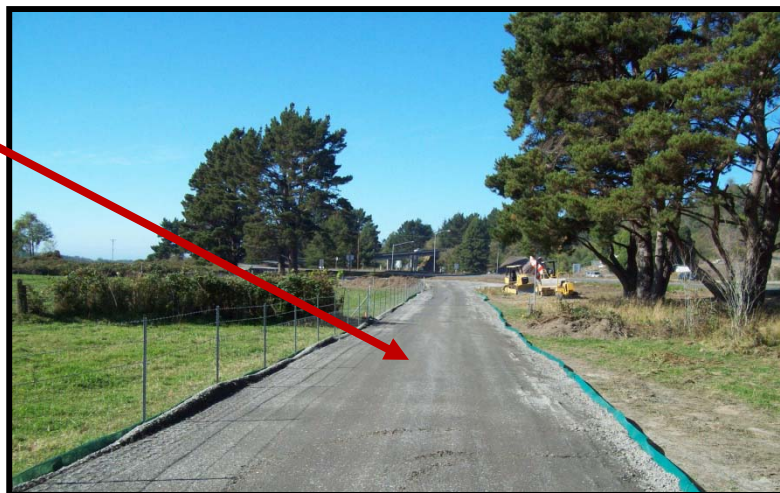
Stabilized construction road.
