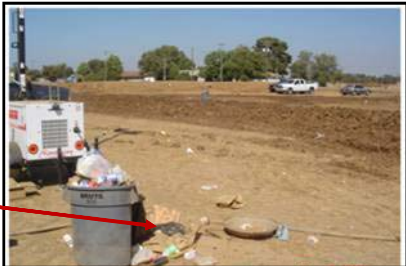
Improperly managed waste receptacle.
