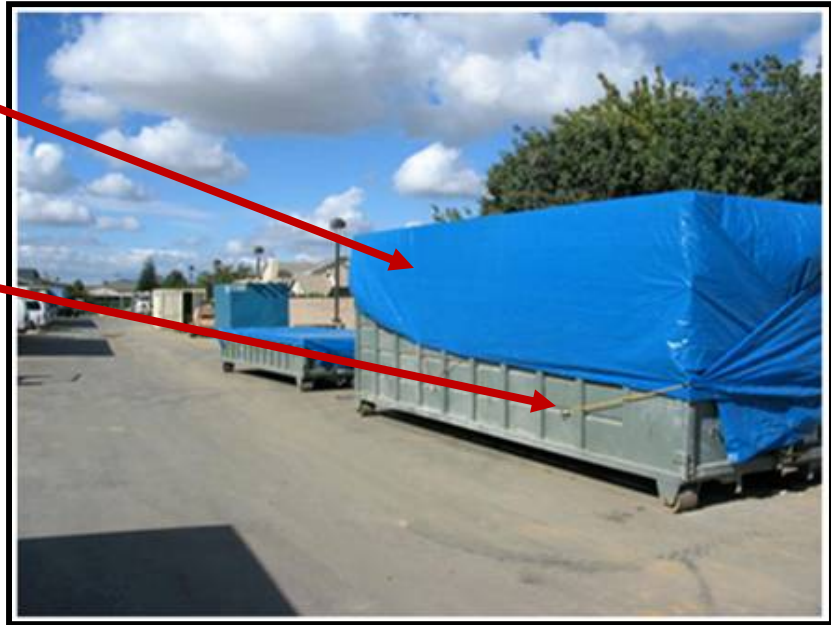
Waste bin with a tarp cover.
