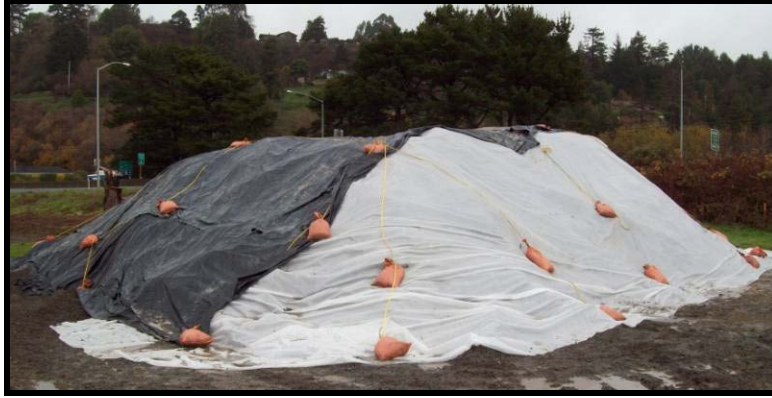
Proper securing of plastic sheeting.
