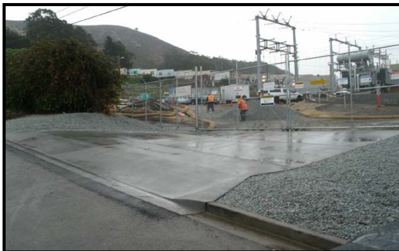
Clean and well maintained construction entrance/exit.
