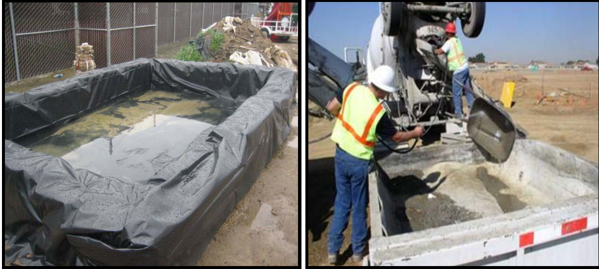
Two alternatives for containing concrete washout water.
