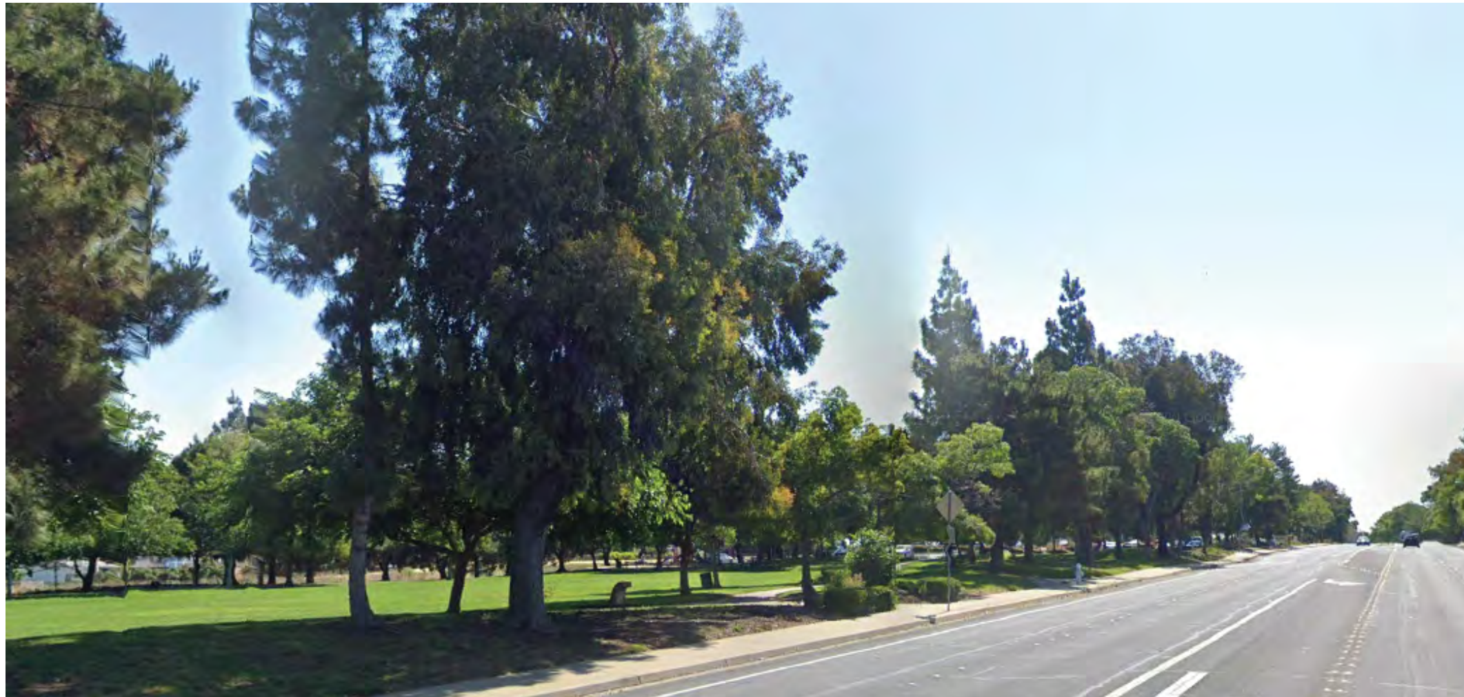
View of Building Site driving East on W. Leland
