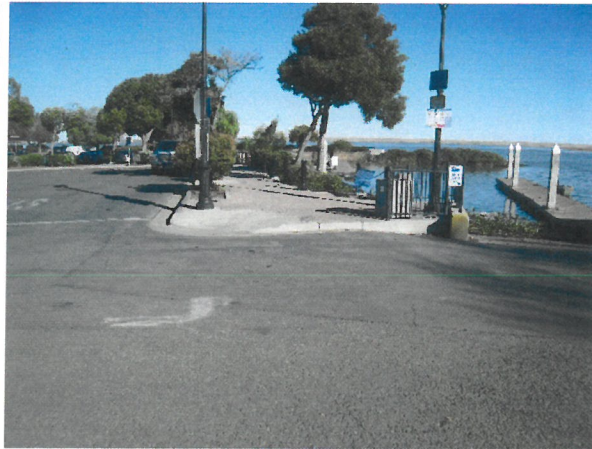
End of existing ADA-compliant path of travel
