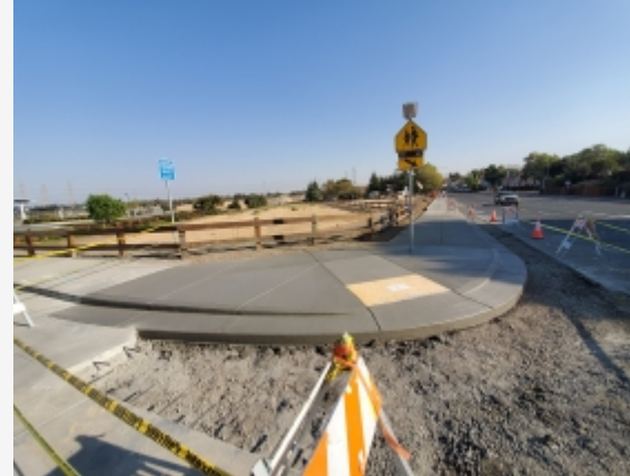
Range Road Sidewalk Widening
