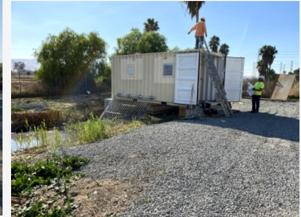
Montezuma Pump Station
