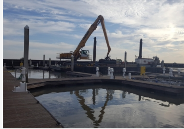
Marina Dredge Project
