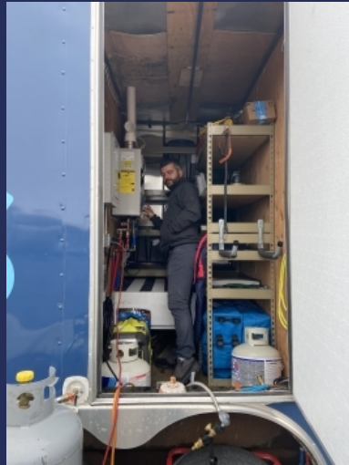
2. Water is heated by a tankless heater.
