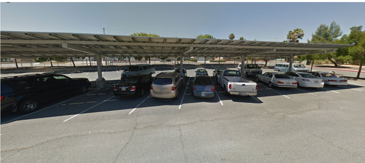
View of parking area at facility
