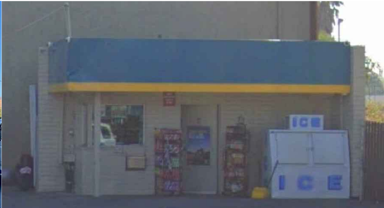
EXISTING KIOSK TO REMAIN (PAINT PER CHEVRON SPEC'S)
