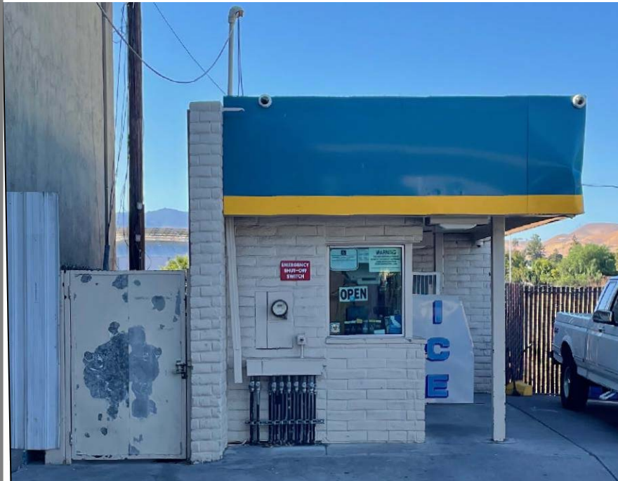
EXISTING KIOSK TO REMAIN (PAINT PER CHEVRON SPEC'S)
