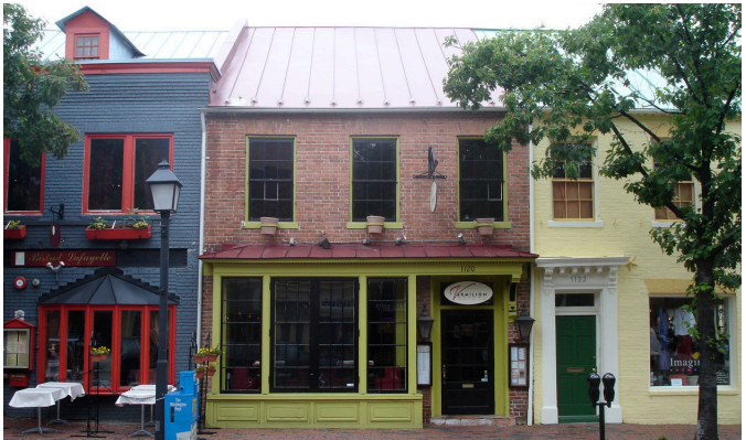
Example of Main Street Building
