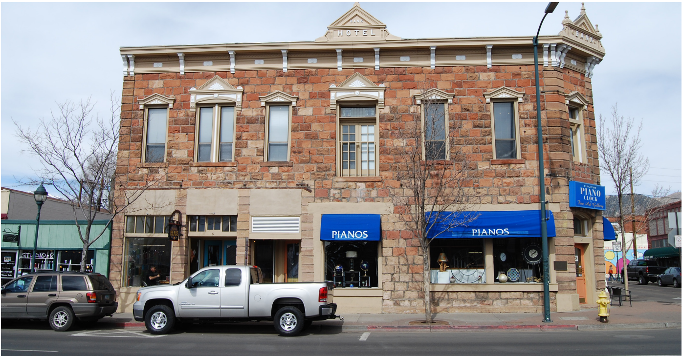
Example of Main Street Building
