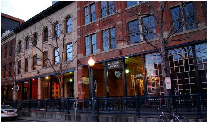
Example of Main Street Building
